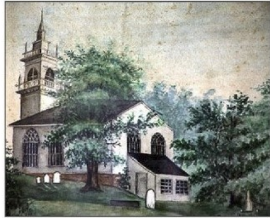
Ralph Leeming's church at Ancaster
